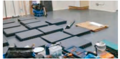
Pic 1. Break down the pallets and allow tiles to acclimatise
