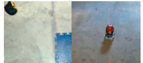
Pic 3. Make sure you keep the tiles square using either a carpenters square, chalk line or laser
